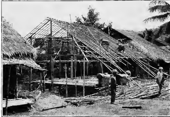
124. LASHING THE ROOF-POLES.
